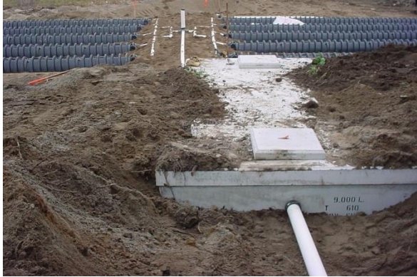
A septic tank and leaching bed
