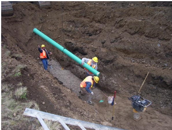
Sanitary sewer pipe installation
